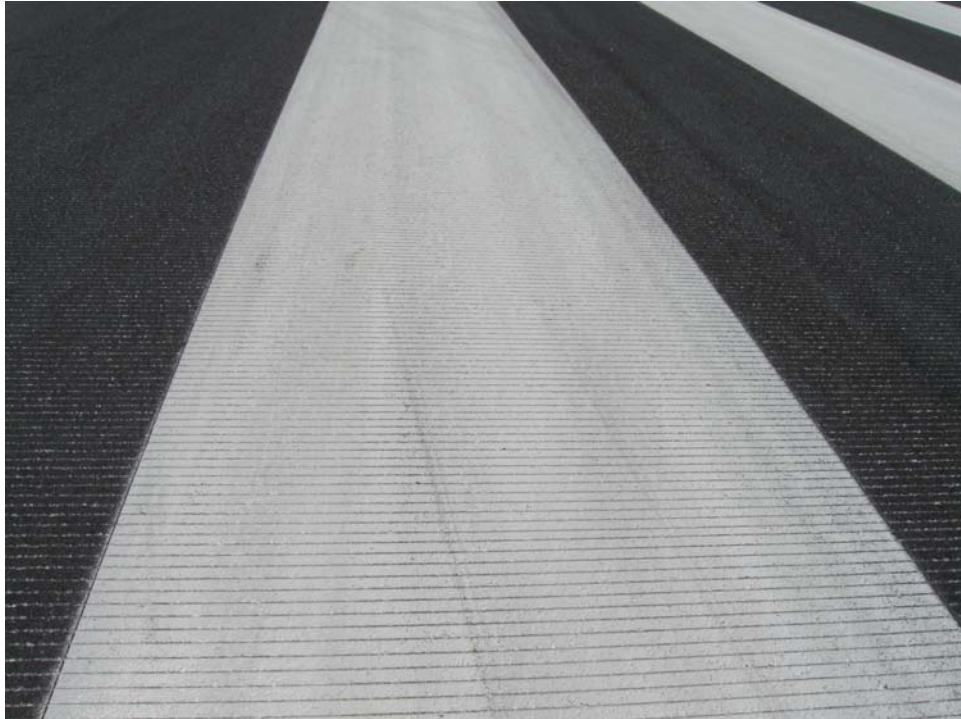
R523MGRA-10C. Satisfactory Paint.
