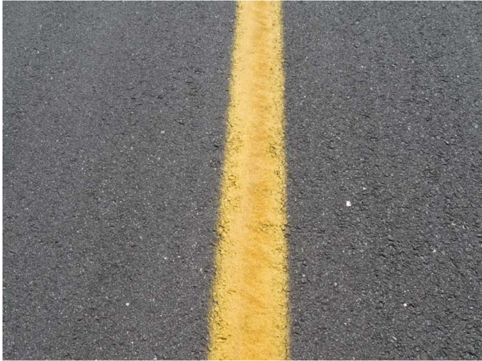
TBMGRA-20. Satisfactory Paint.
