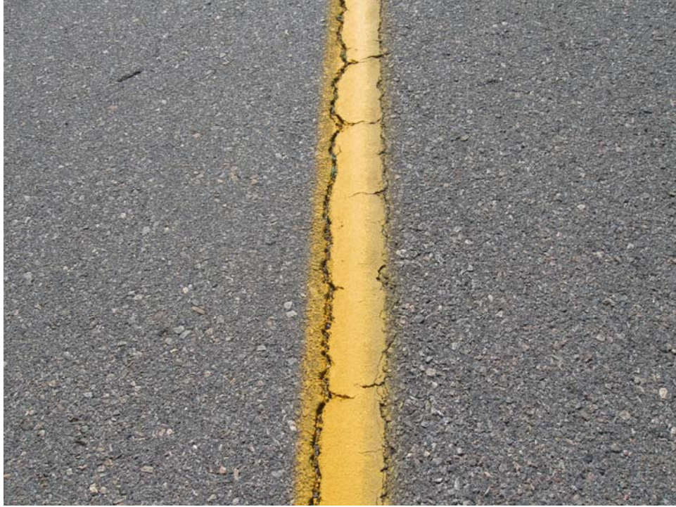
TCMGRA-20. Satisfactory Paint.
