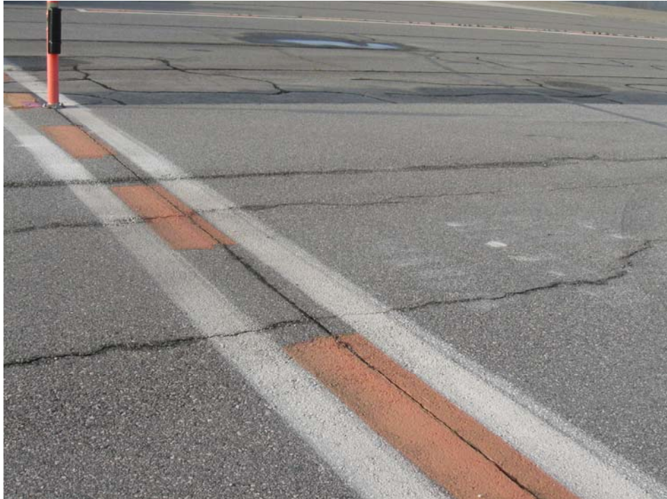
A01MGRA-30. Satisfactory Paint.
