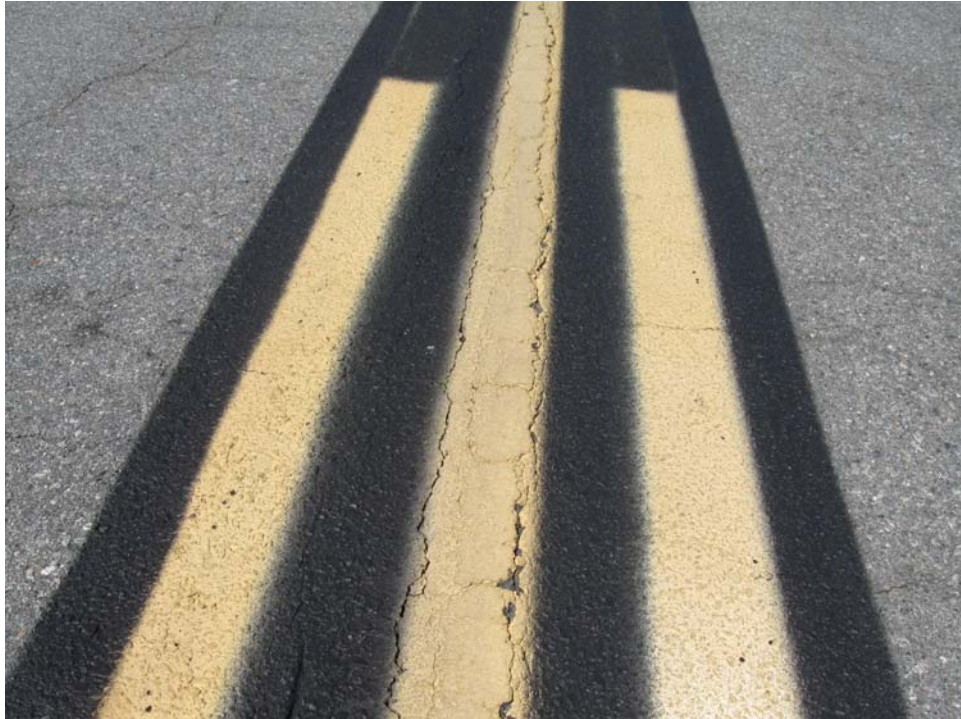
TCMGRA-10. Satisfactory Paint.
