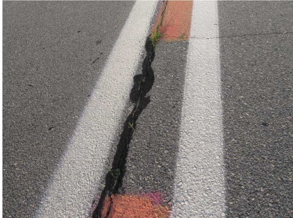
A01MGRA-10. Satisfactory Paint.
