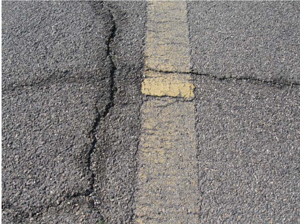
A01MGRA-60. Unsatisfactory Paint.
