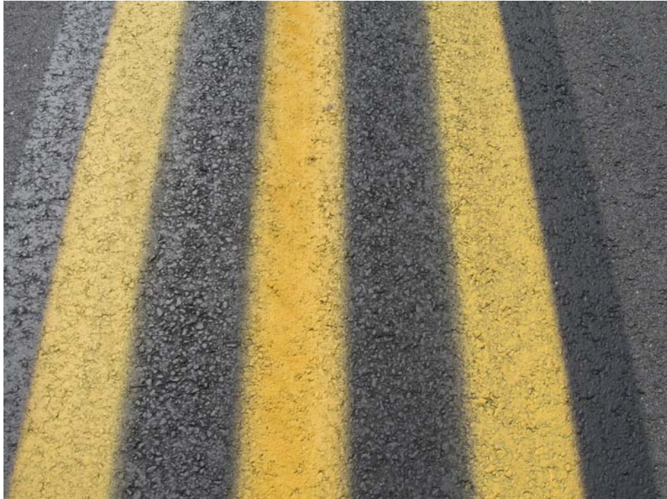
TBMGRA-10. Satisfactory Paint.
